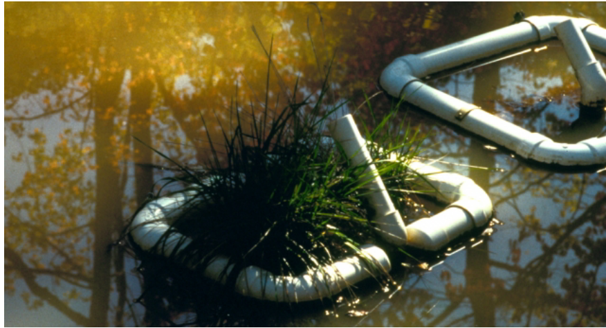
Figure 2-7 Overgrown Vegetation Restricting Movement of Skimmer (Faircloth 2010)
